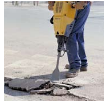
Cutting asphalt
